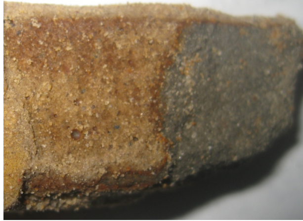
Figure 1: The Sample of Uncoated Silicate Concrete after Testing in a 5% Solution of Hydrochloric Acid.
